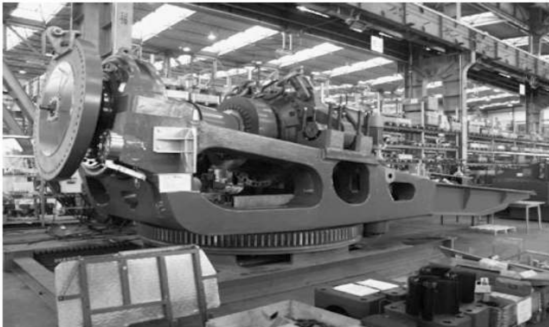
Fig.(1.11): Assembling of a wind turbine with gearbox by NORDEX company (Photo Nordex)
