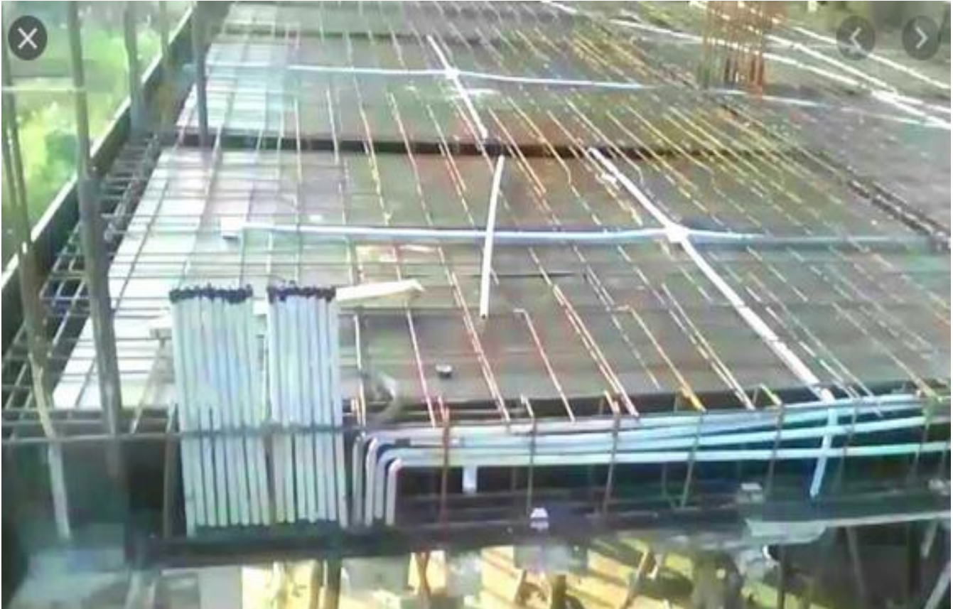
Fig (1.15) Pipe Conducting type
