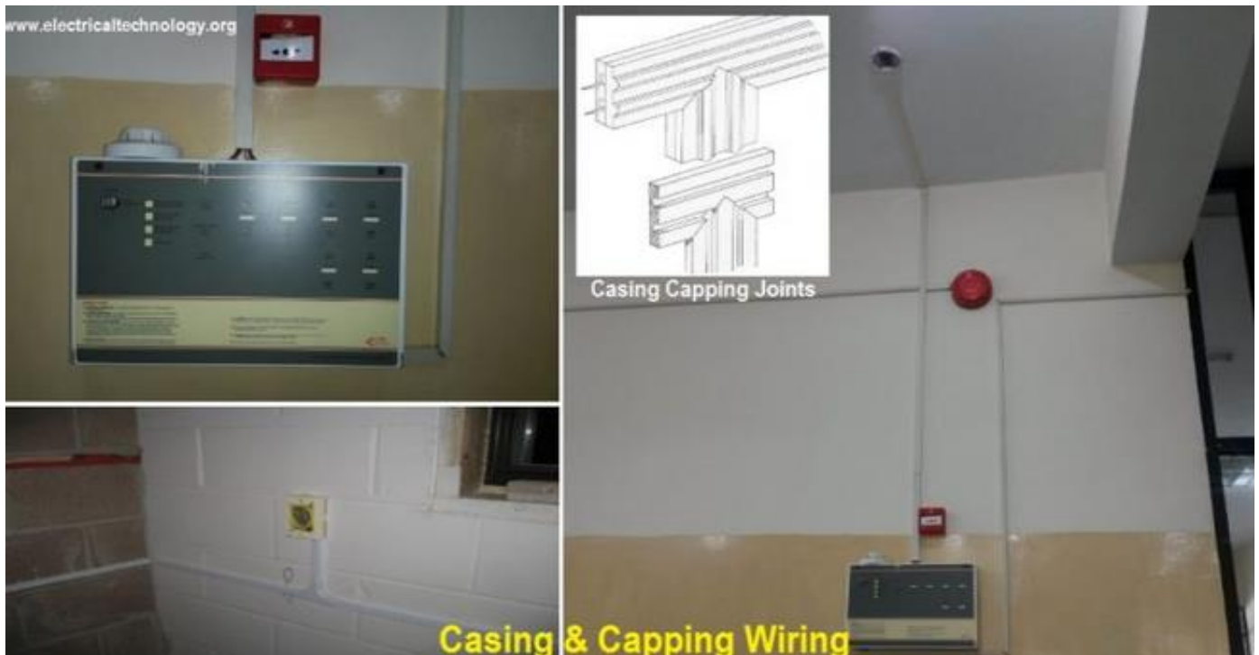
Fig (1 .12) Casing and Capping type
