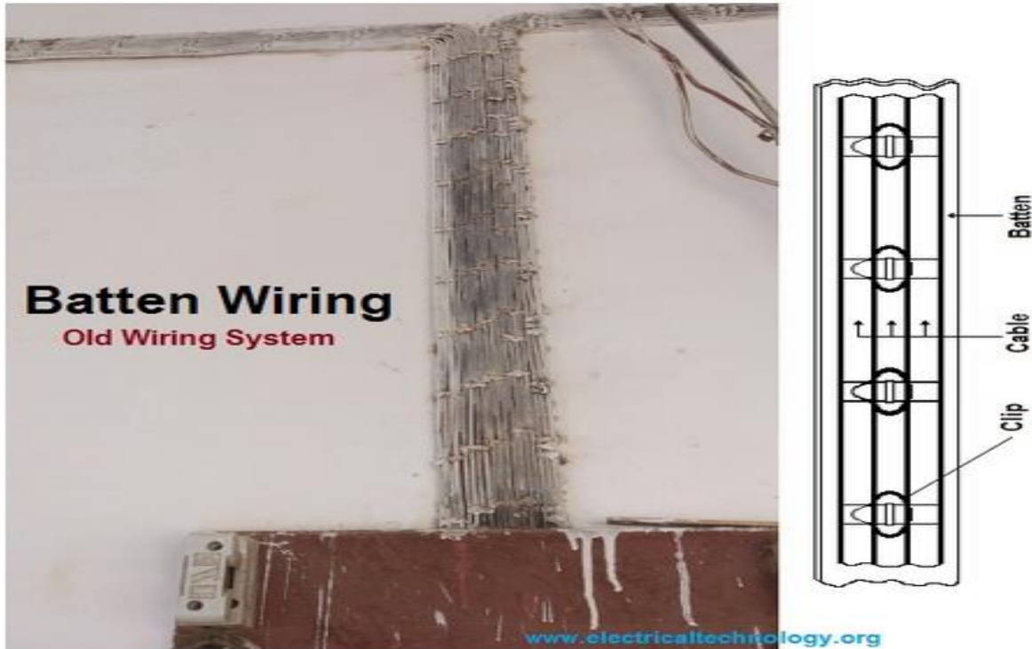
Fig (1.14) Batten Wiring (C.T.S or TRS) system
