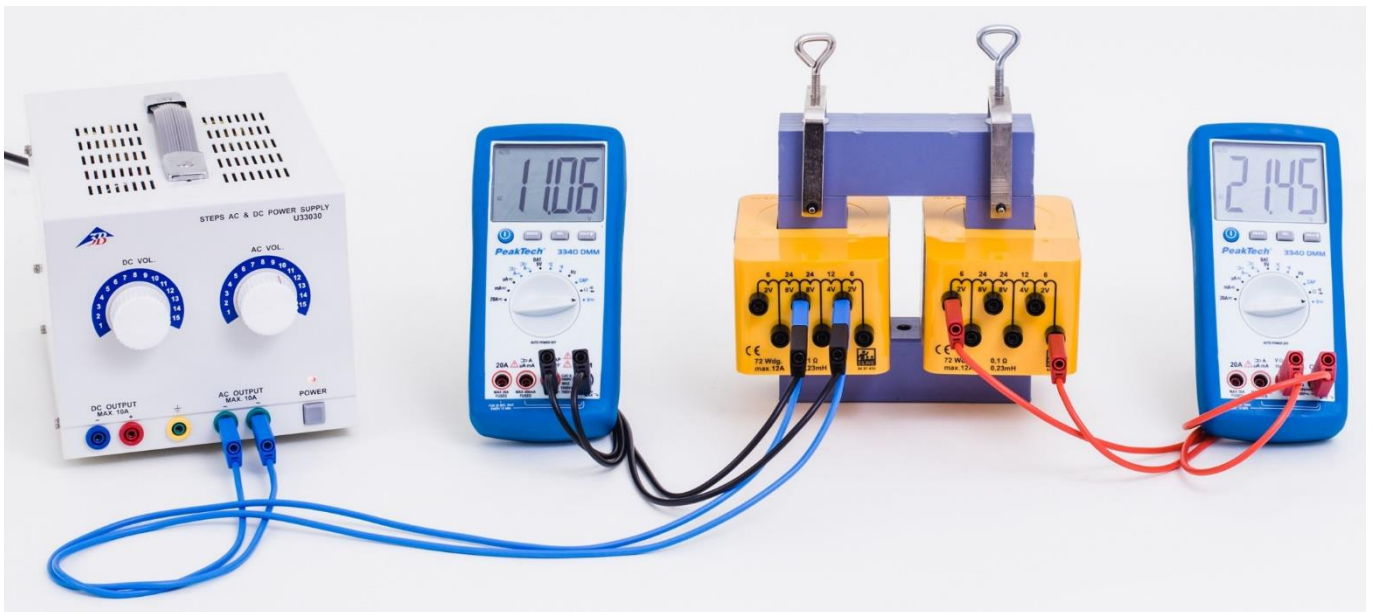
Fig. 1: Set-up for measuring open-circuit voltage as a function of primary voltage.
