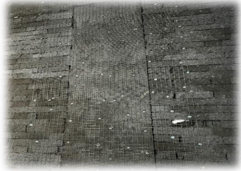
Figure 2.10 show BRC on the wall in case having joints.
