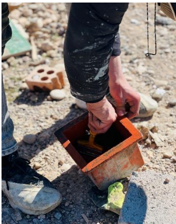
Figure 2.17 mould apply oil
