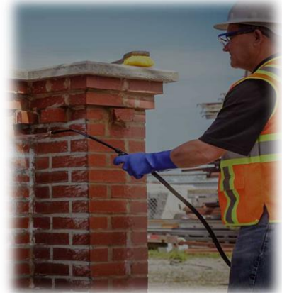
Figure 2.6 process of curing wall
