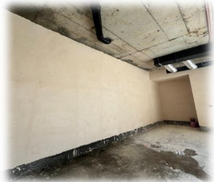
Figure 2.8 process of internal plastering during finishing first layer
