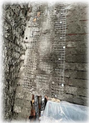
Figure 2.11 double BRC used because mechanical works on the wall.
