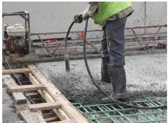
Figure 2.24 the process of using vibrator in fresh concrete
