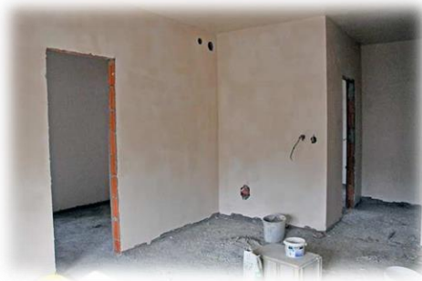
SFigure 2.13 demonstrate first layer of internal plastering.
