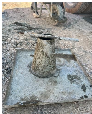
Figure 2.19 Prepare a slump cone
