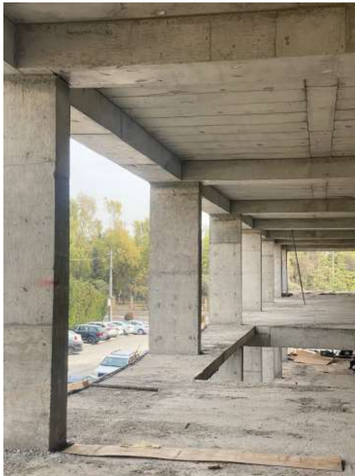
Figure 4-6: Picture of removed columns from the other floors
