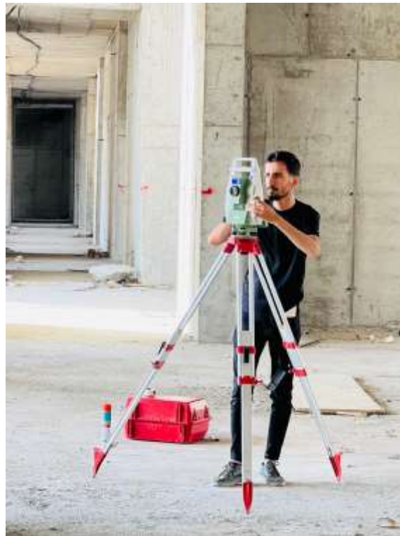
Figure 3-13: Measuring by total station Leica TS15
