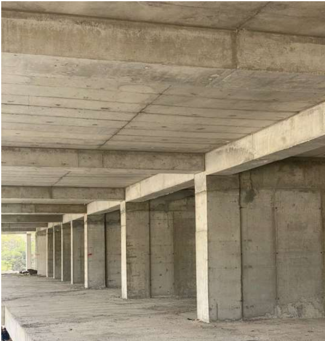
Figure 4-10: Show the concreted beams and slab
