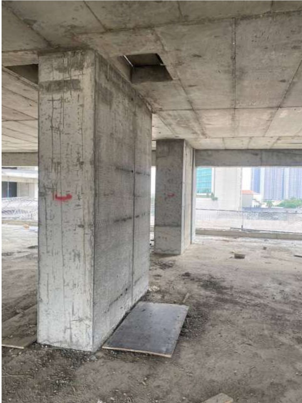
Figure 4-8: Show the concreted shear walls
