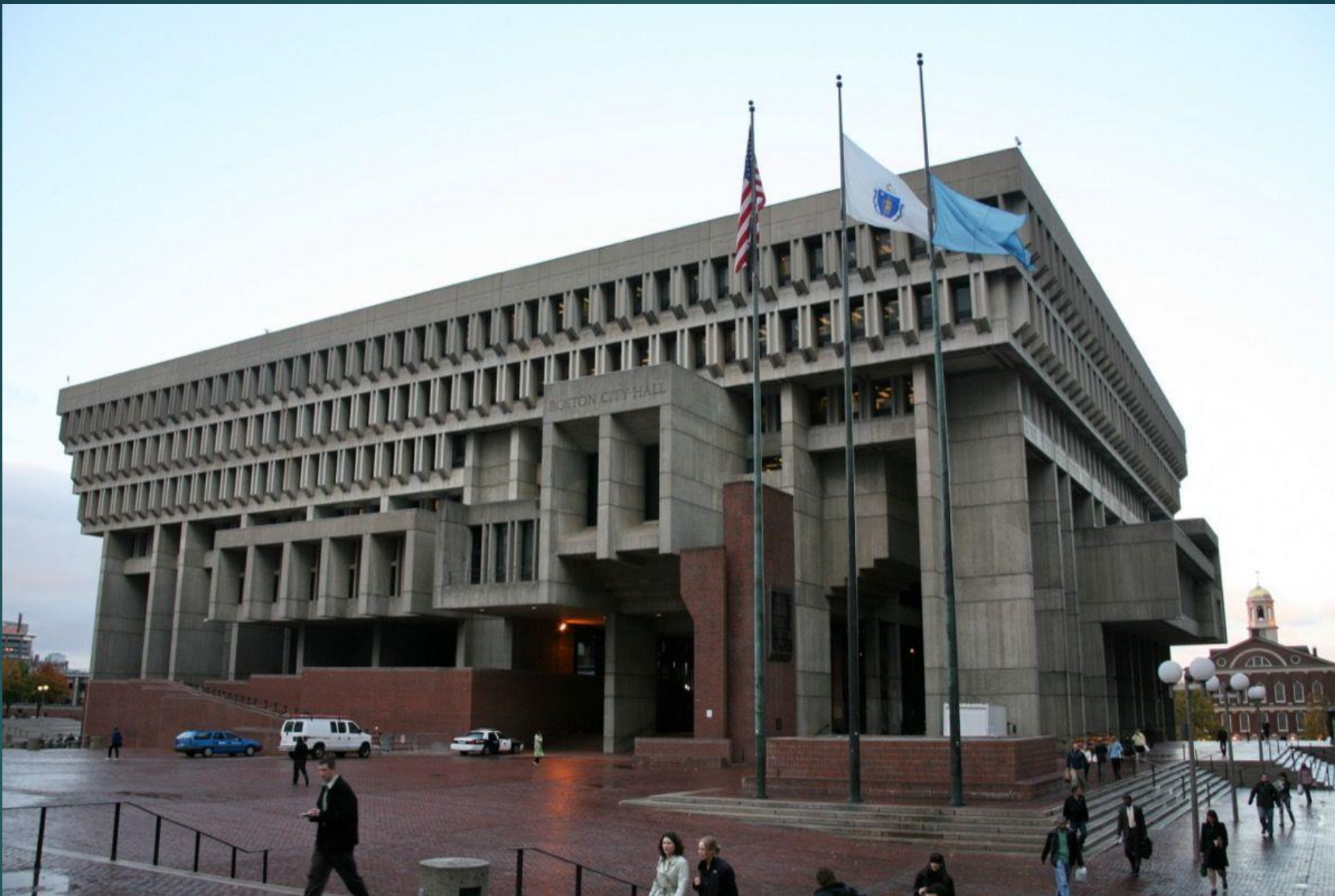
Boston City Hall, Boston, MA, 1968 Varied exterior forms delineate different functions (such as the council chamber and mayor's office), while deep-set window openings create a highly textured façade.
