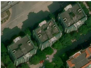
Regular Orthophoto showing the relief of the building.
