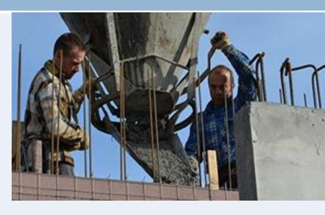
During the concrete filling the verticality of the wall is checked and corrected if necessary. When the concrete is dry enough, the scaffolding can be removed.
