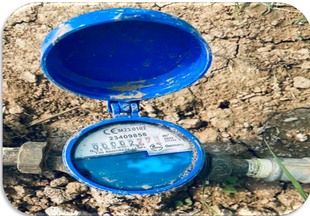
Fig. 5 Water meter for calculate volume of water in the RDI system.
