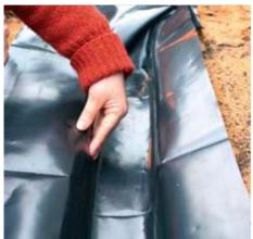
3-Line the rill with the liner, smoothing out any creases. Trim the liner at the reservoir end so that it drapes over the rim. Leave 8 in (20 cm) surplus along the other three sides.
