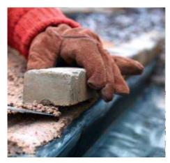
4-Edge the rill with bricks on three sides (not the reservoir end). Bed bricks on a 1 in (2 cm) layer of waterproof mortar, making sure that it doesn't fall into the rill. Mortar between the bricks.
