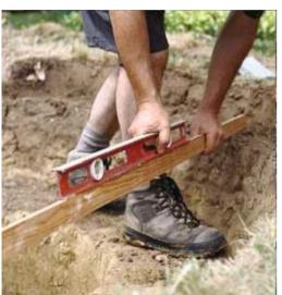
4- Use a level placed on a straight piece of wood to check that the ground around the top of the pond is level. Remove any loose soil and all large or sharp stones from the sides and bottom of the pond.
