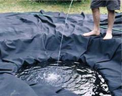
6-Center the liner over the hole, letting it slide down under its own weight into the base. Leaving plenty of surplus around the rim, pleat the liner to help fit it to the shape of the pond. Fill with water.
