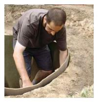
5- To protect the liner, line the sides and base of the pond with pond underlay. If using old carpet underlay, beware stray tacks. On stony soils, spread a 2 in (5 cm) layer of sand over the base first.
