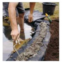
7-When the pond is full, trim the surplus liner leaving 18 in (45 cm) around the rim. Pleat the excess liner so it lies flat and bury the edges in the ground. Lay a bed of waterproof mortar for the edging stones.
