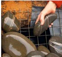
6-Cover over the pipe in the rill with a level bed of gravel. Place a metal grille over the reservoir and top with cobbles. If you sit them on a sheet of permeable fabric it will stop debris falling into the water.
