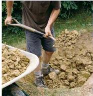
2- Before you start digging, skim off any sod for reuse elsewhere. Keep the fertile topsoil (which you can also reuse) separate from the subsoil. Loosen compacted subsoil with a pickax.
