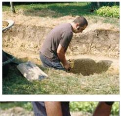
3- Dig out the pond to a depth of 18 in (45 cm). Make the sides gently sloping. Leave a shelf 12–18 in (30-45 cm) wide around the edge, then dig out the center to a further depth of 18 in (45 cm).
