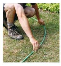
1- Use a hose to mark the outline of the pond. Aim for a curved, natural shape without any sharp corners. To prevent it freezing solid in winter, a section of the pond must be at least 18 in (45 cm) deep.
