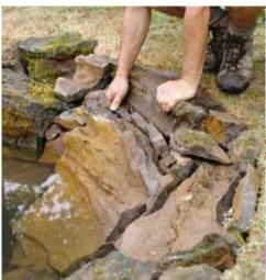
8-Bed the edging stones into the mortar, overhanging them by 2 in (5 cm) to hide the liner. When positioning vertical stones, stand them on a piece of rolled-up surplus liner to protect the liner from being worn.
