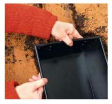
2-Line the rill with sand, compacting it with a piece of wood. Use a level to check the base is flat. Dig a hole at one end and insert the reservoir—check that the rim is level with the base of the rill.
