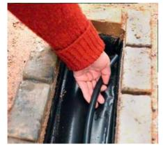
5-Place the pump in the reservoir. Push the pipe on to the pump outlet, run the pipe along the length of the rill, and cut it to fit at the far end. Fit a filter on the free end of the pipe to prevent blockages.
