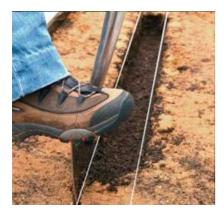
1-Clear and level the site. Mark out the length and width of the rill with pegs and string. Dig out the area to a depth of 6–8 in (15–20 cm). Cut a shallow shelf all around the rill for the brick edging.
