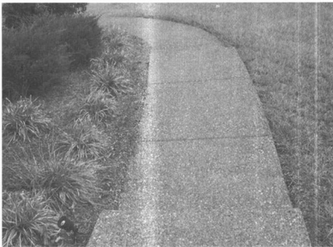
Figure 6-18 Exposed Aggregate Pea gravel embedded into concrete.
