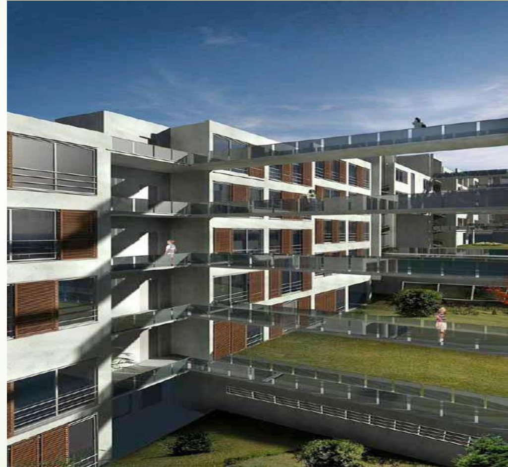
A view from the interior garden, Block Design 363
