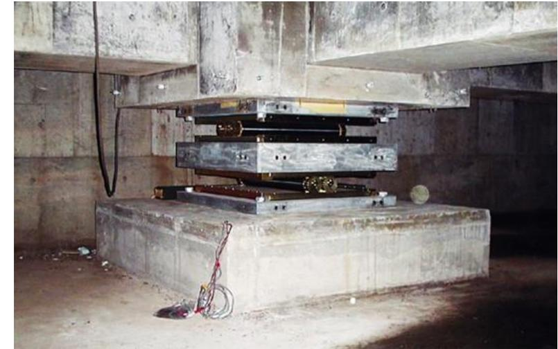
Spherical Sliding Bearing
