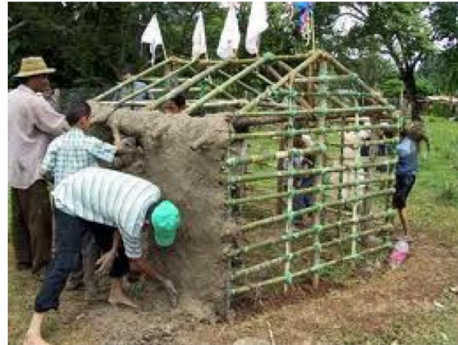
Mud being Plastered to wooden Framework
