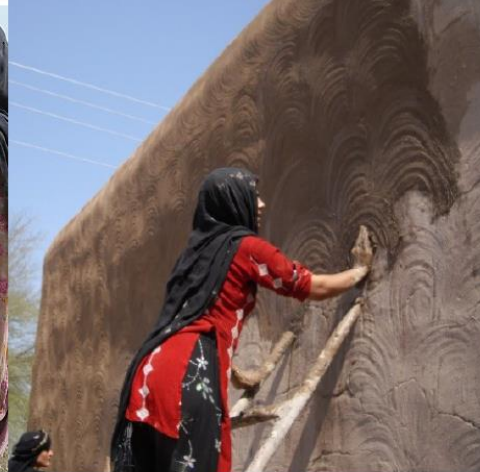
Mud being Plastered to wooden Framework
