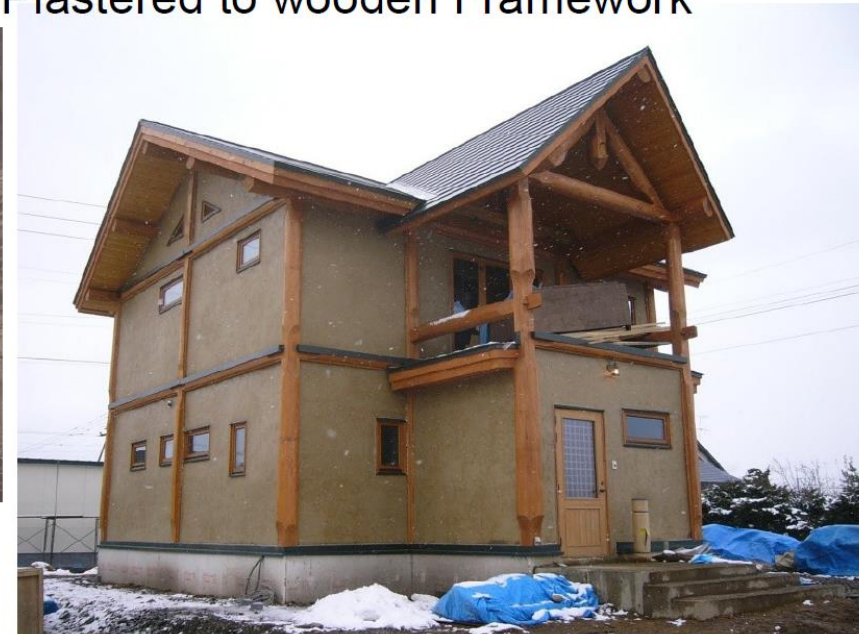
Mud being Plastered to wooden Framework
