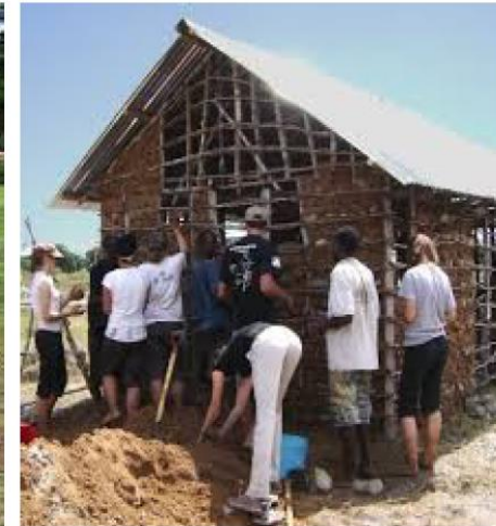
Mud being Plastered to wooden Framework
