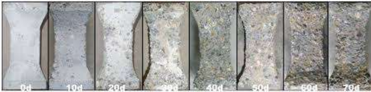
Figure.11 ( change of concrete due to acid rain effects over time)
