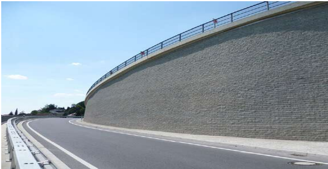
Figure 1.11 highway Retaining wall
