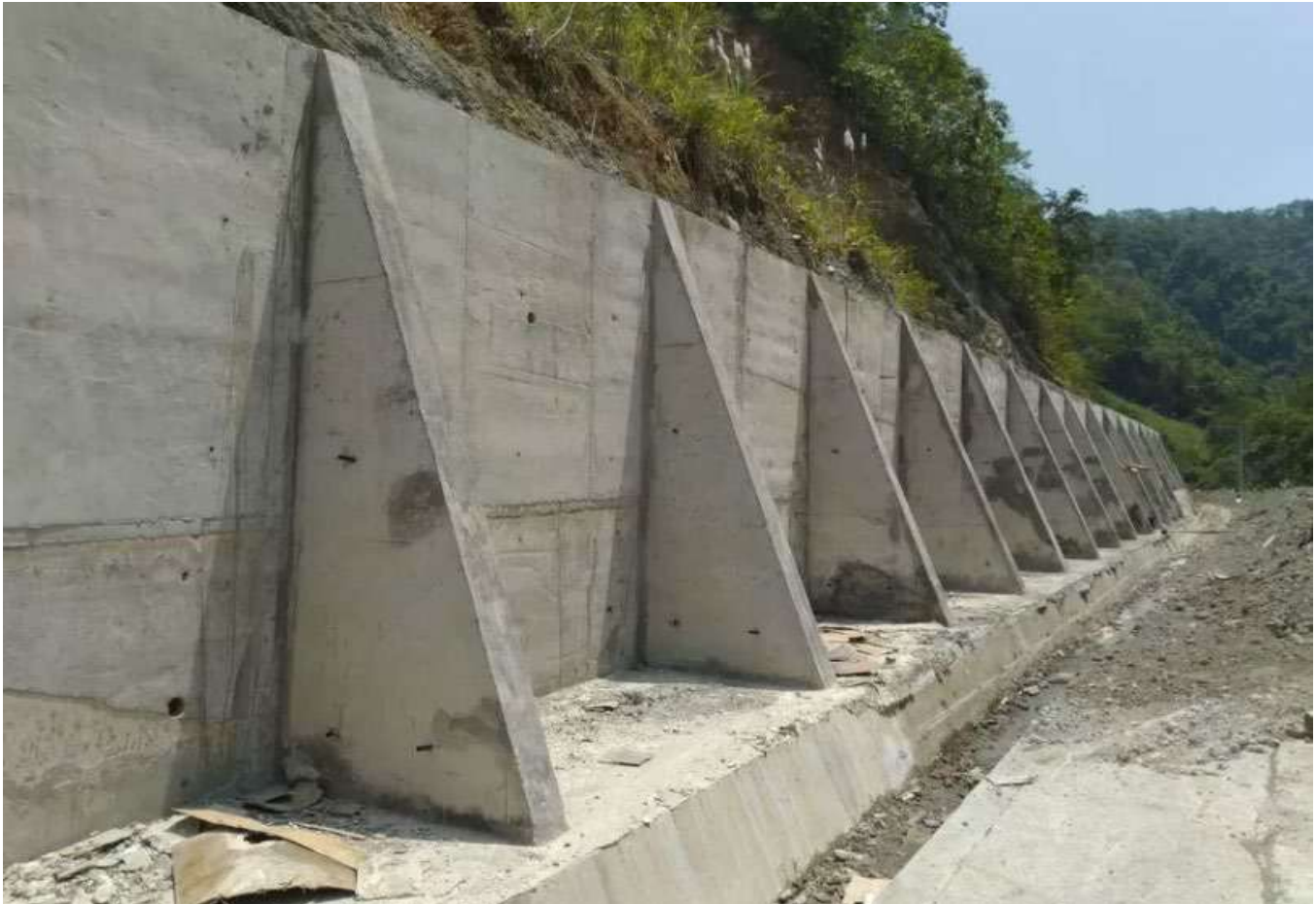
Figure 2. Buttress Retaining Wall
