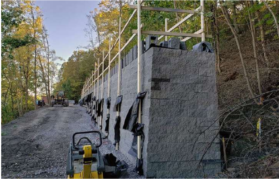
Figure 1.8 retaining wall for protection rock and soil falls
