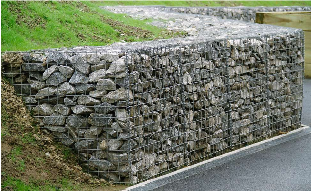
Figure 2.7 Gabion Retaining Wall
