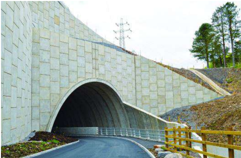
Figure 1.13 tunnel portal retaining wall
