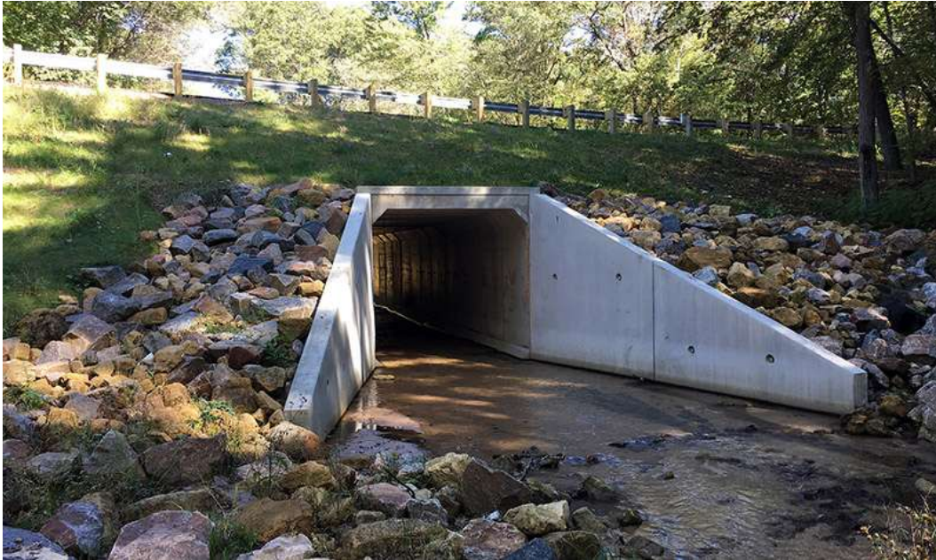
Figure 1.12 culvert retaining wall
