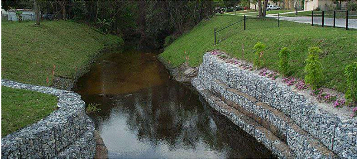
Figure 1.10 Gabion River stream and coastal erosion control.
