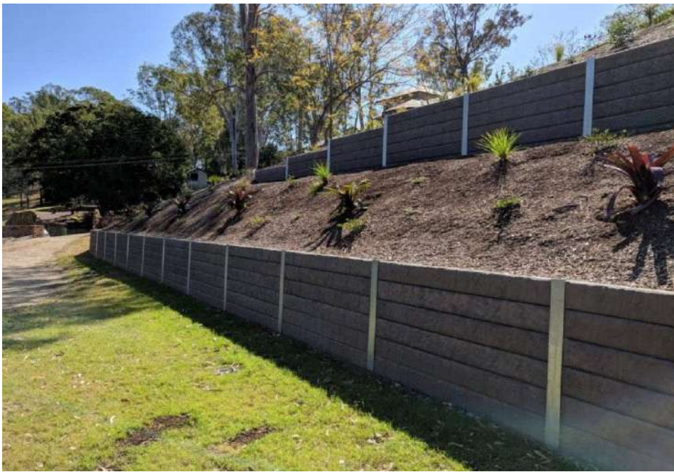
Figure 1.1 retaining wall supports a building side slope
