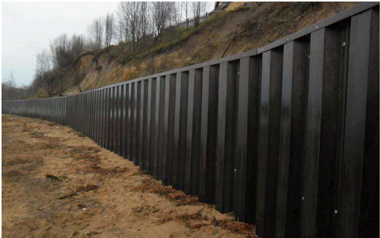
Figure 2.2 sheet pile retaining wall
