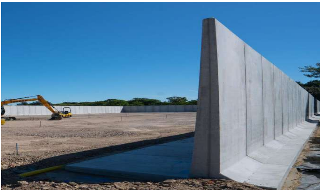
Figure 2.3 cantilever retaining wall
