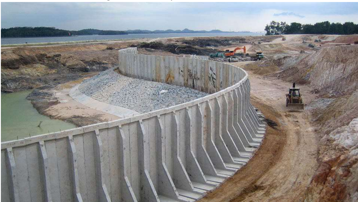
Figure 2. Counter Retaining Wall
