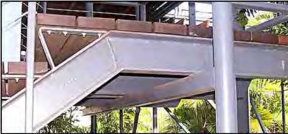
Steel stairs - Transition from string to landing.
