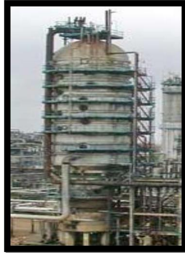
Vacuum Distillation Tower
