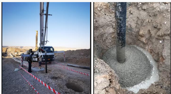
Fig. Plastic concrete placing.
