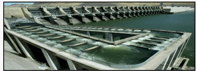
Fig. Fish ladder system.
