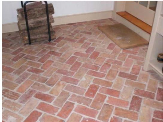
4- **Paving bricks** are used as a paving material for roads, sidewalks, patios, drive ways, and interior floors. Paving bricks available in different colors such as red, gray, or brown and typically they are abrasion resistance and could be vitrified.
