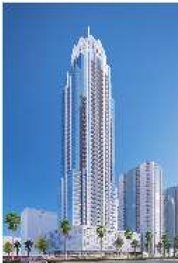
High- Rise Building (skyscraper)/ Zanyary tower-Erbil
