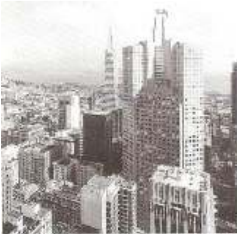
(a) View of hotel (building on the right)
