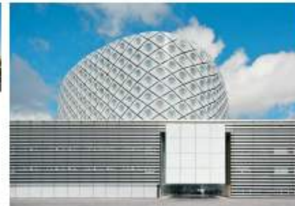
Rey Juan Carlos Hospital (2008) designed with the general layouts (Access to emergency Department)
