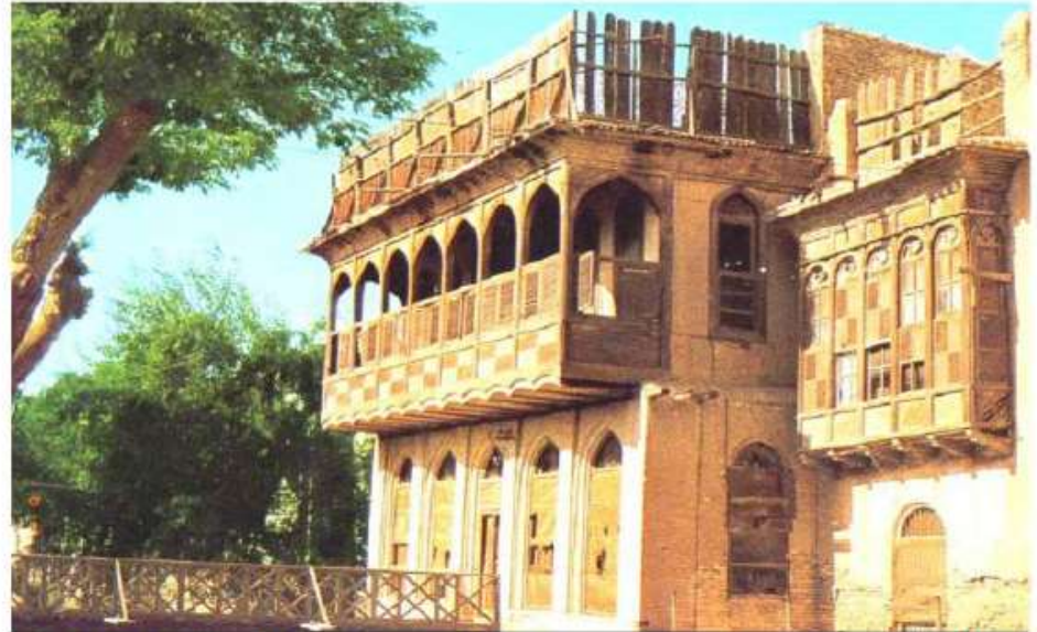
Fig. 3 (left) Grilled external windows mashrabiya is one of the distinguished elements used for privacy and penetration of solar radiation, picture for traditional house in Basra-Iraq
